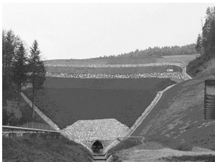
Fig.2. Jazbec pile after contouring and cover construction of the eastern slope (2007), at the bottom the outlet of the culvert draining to the Brebovčica creek.
