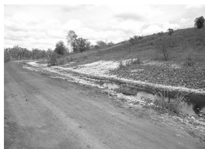
Fig.3. Waste rock dump infiltration : monitored infiltration rate (left), White's WRD in July 2007 (right) – note the active seepage flow and characteristics (photo G M Mudd).
