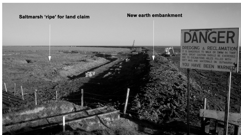
Figure 19 Erection of an earthen embankment, southwest shore of the Wash in the late 1970s
