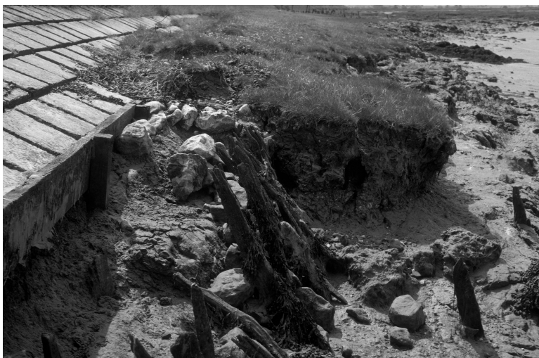
Figure 42 Eroding saltmarsh undermining a sea wall, Essex
