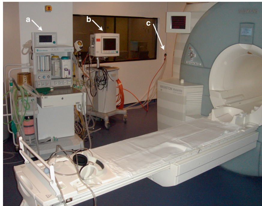
Fig. 2 Cardiovascular MR set-up for paediatric general anaesthetic cases. View of the MR scanner room showing the anaesthetic machine (a) and monitoring equipment (b). Ventilation tubing and leads from both pieces of equipment pass through a small opening in the wall (c) into the control room, so that the anaesthetist can control breath-holding and monitor the patient from within the control room
