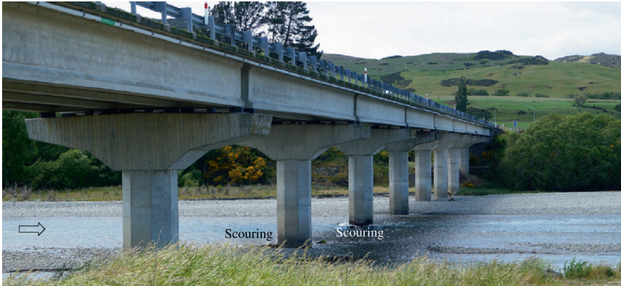
Fig. 10.18 Scour taking place at bridge piers in a field condition. Photograph by the author
