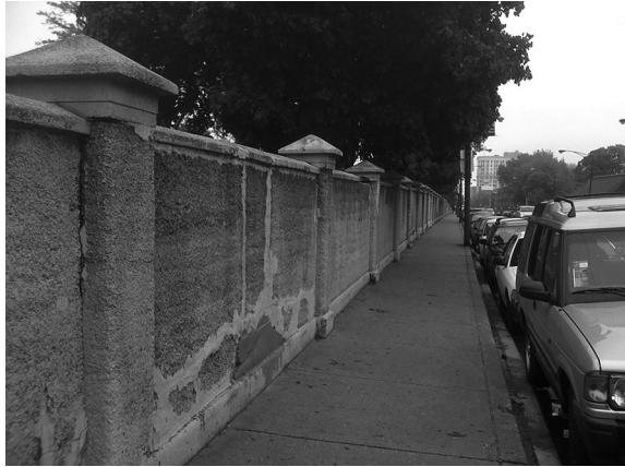
Fig. 8.9 Reinforced pervious concrete walls
