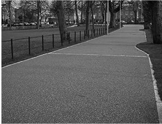
Fig. 16.6 Resin based pavement path (McCormack 2010)
