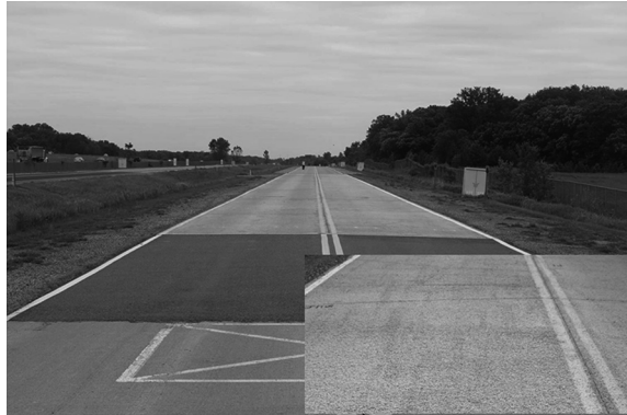
Fig. 8.7 Pervious concrete overlay for noise reduction
