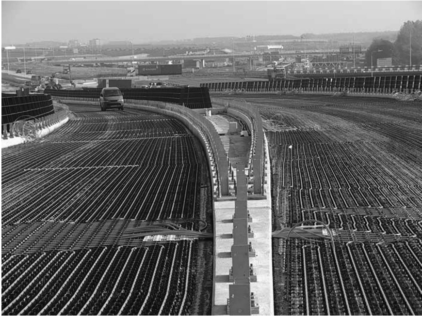
Fig. 18.8 Asphalt solar collector system under construction on a bridge in Rotterdam (de Bondt 2003)
