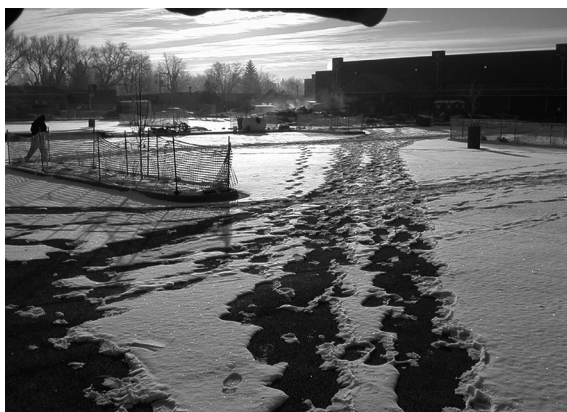
Fig. 8.6 Reduced slip and fall potential of snow-covered pervious concrete
