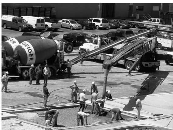
Fig. 8.5 Pervious concrete construction using a belt placer
