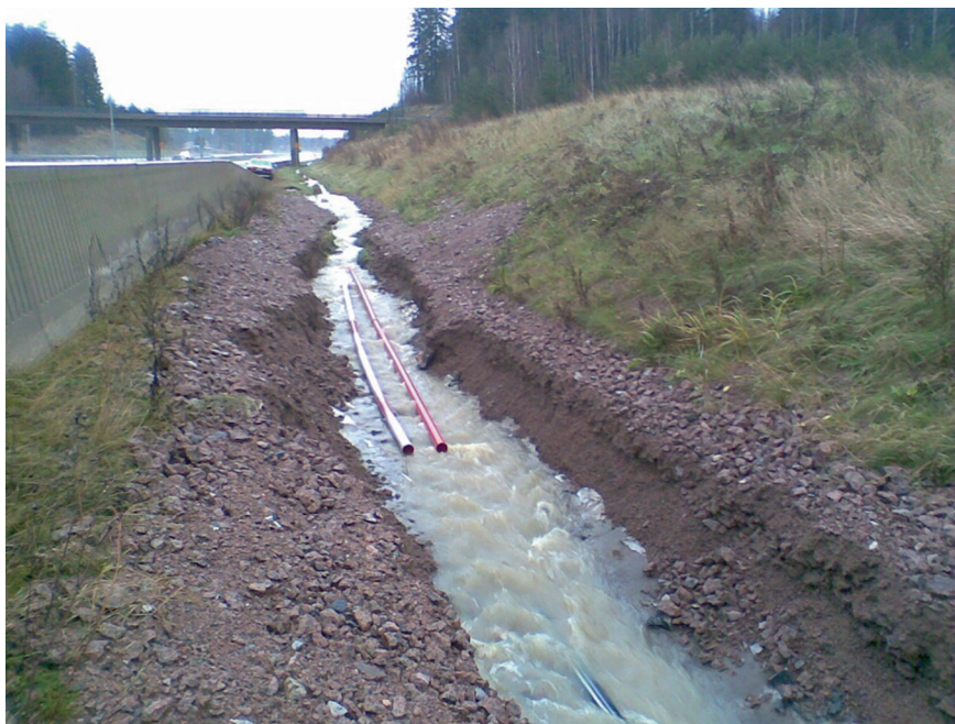
Fig. 4.6 Excessive run-off/seepage eroding the top of a drain following heavy rainfall (courtesy of Antero Nousiainen)
