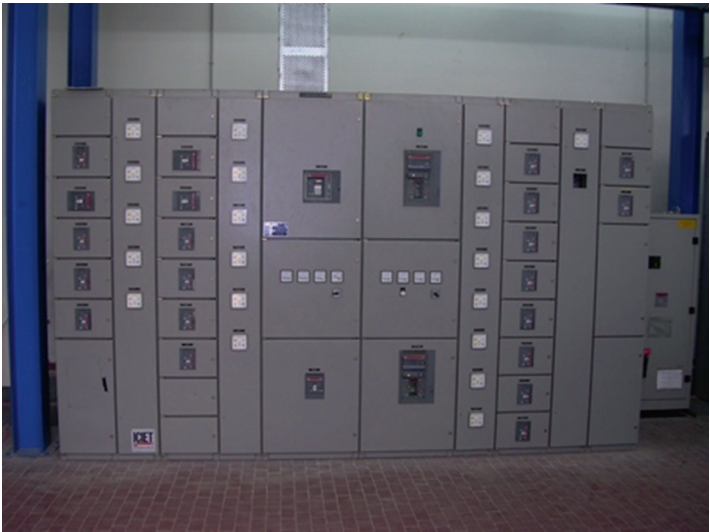
Fig. 12.16 Example of general switchboard panel
