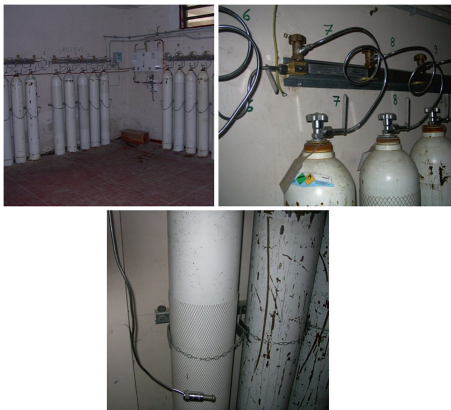
Fig. 12.10 Example of oxygen cylinders – detail of anchorage
