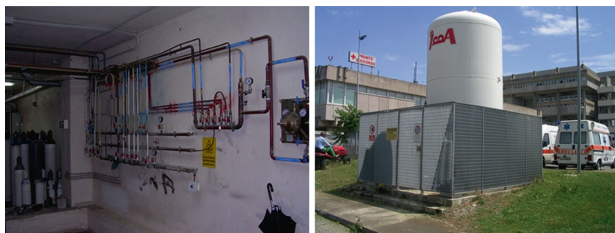
Fig. 12.11 Examples for distribution lines ( left ) and for oxygen bottle tank ( right )
